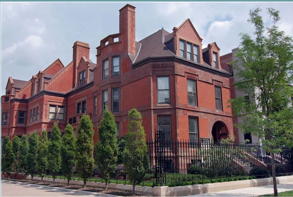
1919 South Prairie Avenue - After
