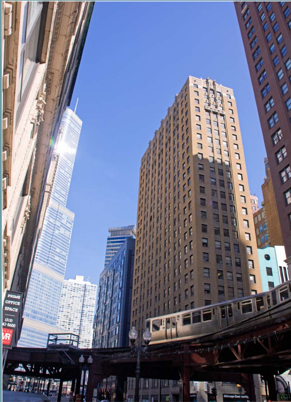
203 North Wabash Avenue - Commercial
